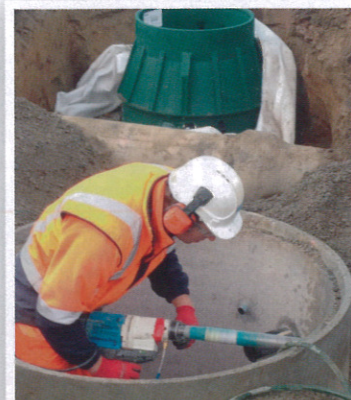
Burton Hawkin of Tru-Line Drainage Ltd, a subcontractor of McConnell Dowell, installing a manhole as part of the vacuum system in Golf Links Road. A partly installed collection chamber is in the background.
