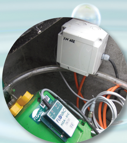
Monitor Operation of the Vacuum Valve
