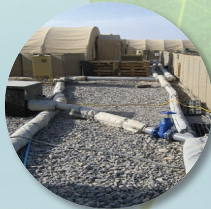
Pipework can remain above ground for easy mobilisation
