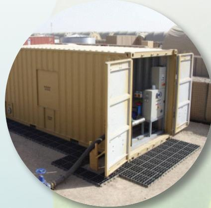
Containerised vacuum pump stations integrated with wastewater treatment plants
