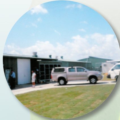
Vacuum Pump Station
