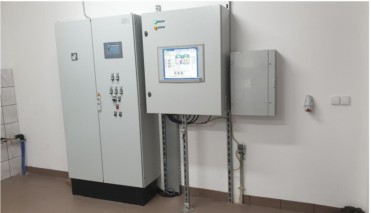
Imielin vacuum pumping station control cabinet and cable monitoring control panel
