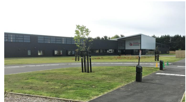
Marshlands School with Collection Pits and Flovac Pillars
