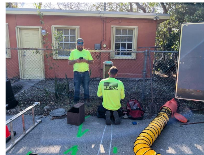
Installation of the monitoring system
