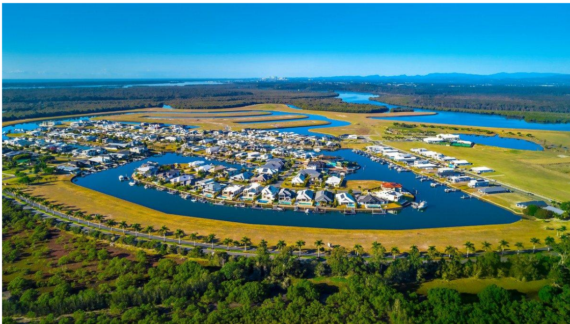
Calypso Bay, Queensland — canal residential development surrounded by waterways. Water table at or near surface throughout.
