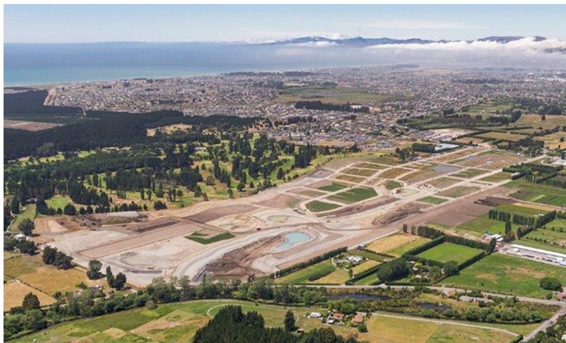
Prestons Park during construction — 203 hectares of flat Canterbury plains land, north-east Christchurch. High water table throughout.
