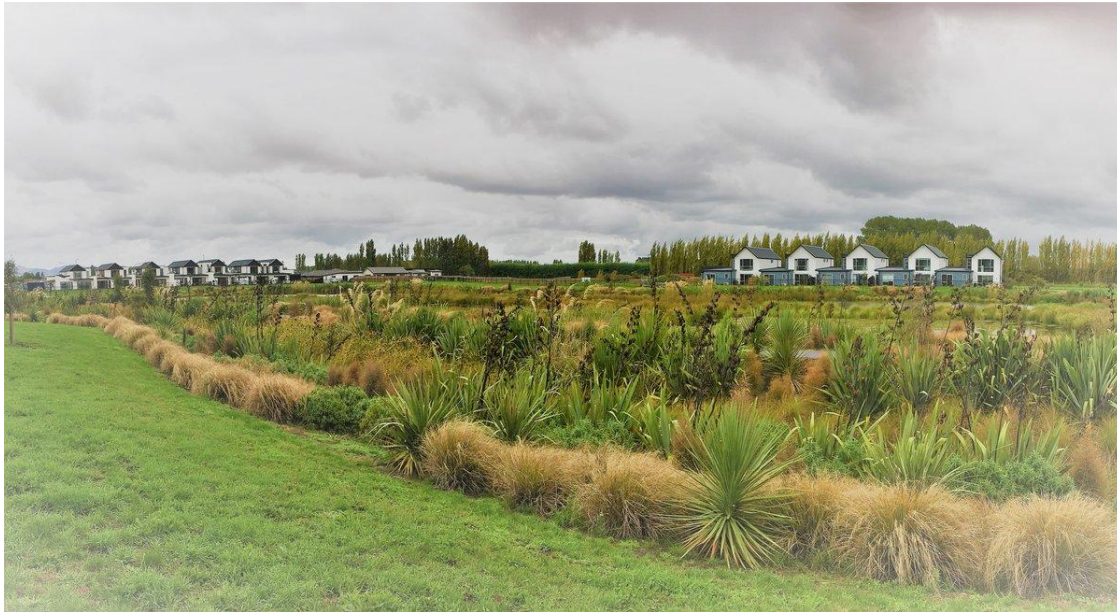
Prestons Park completed — flat terrain, shallow water table, post-earthquake ground conditions that made deep gravity excavation impractical.
