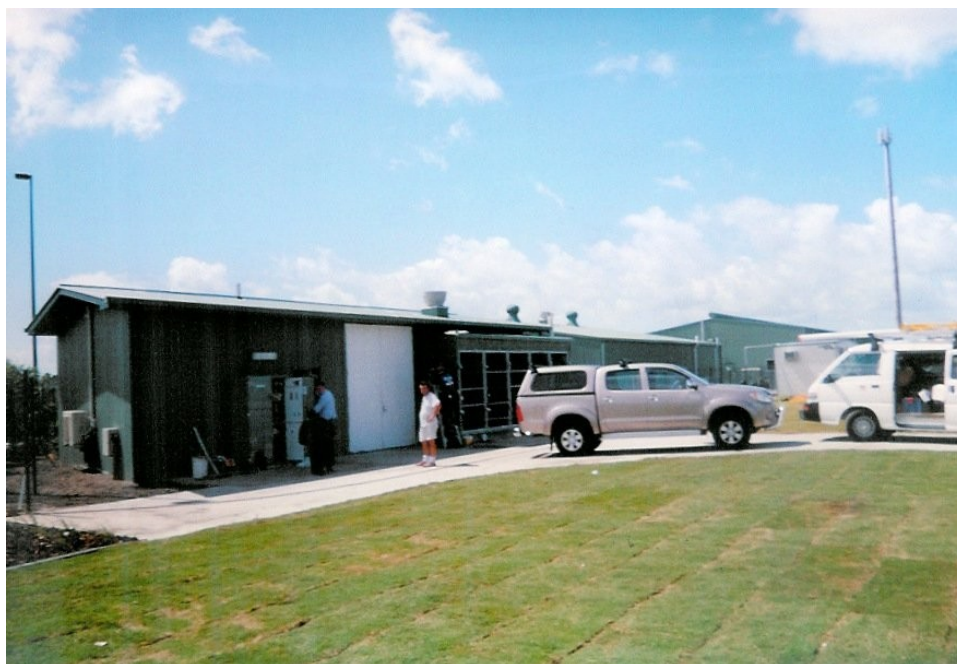
Pacific Harbour Vacuum Pump Station, Queensland — a single facility that replaced 18 gravity pump stations. All collection system energy, maintenance obligations, and operational monitoring consolidated into one location.
