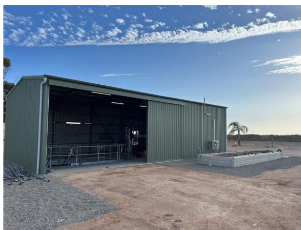
The Fishermans Bay Vacuum Pump Station — all plant for 400 dwellings in one building.
