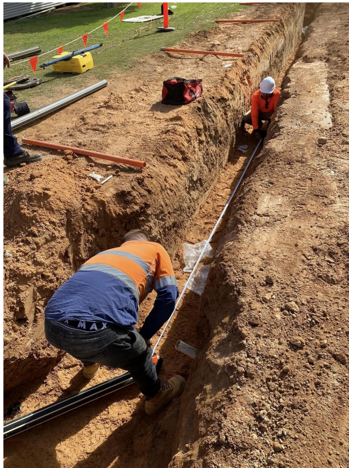
Vacuum reticulation installation at shallow depth in sandy coastal soils typical of the Fishermans Bay site. In a gravity system, these same soils create a direct pathway for groundwater infiltration into the sewer network.
